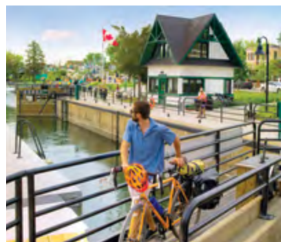
↑ ÉCLUSE NO. 9, PARCS CANADA
