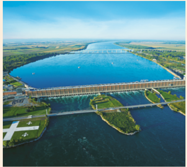
→ BEAUHARNOIS HYDROPOWER GENERATING STATION ©HYDRO-QUÉBEC
