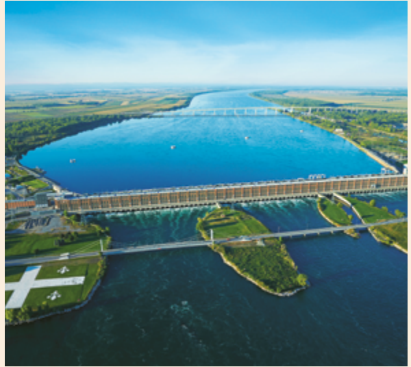
→ BEAUHARNOIS HYDROPOWER GENERATING STATION ©HYDRO-QUÉBEC
