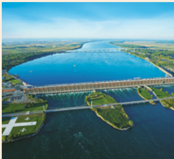
→ BEAUHARNOIS HYDROPOWER GENERATING STATION ©HYDRO-QUÉBEC
